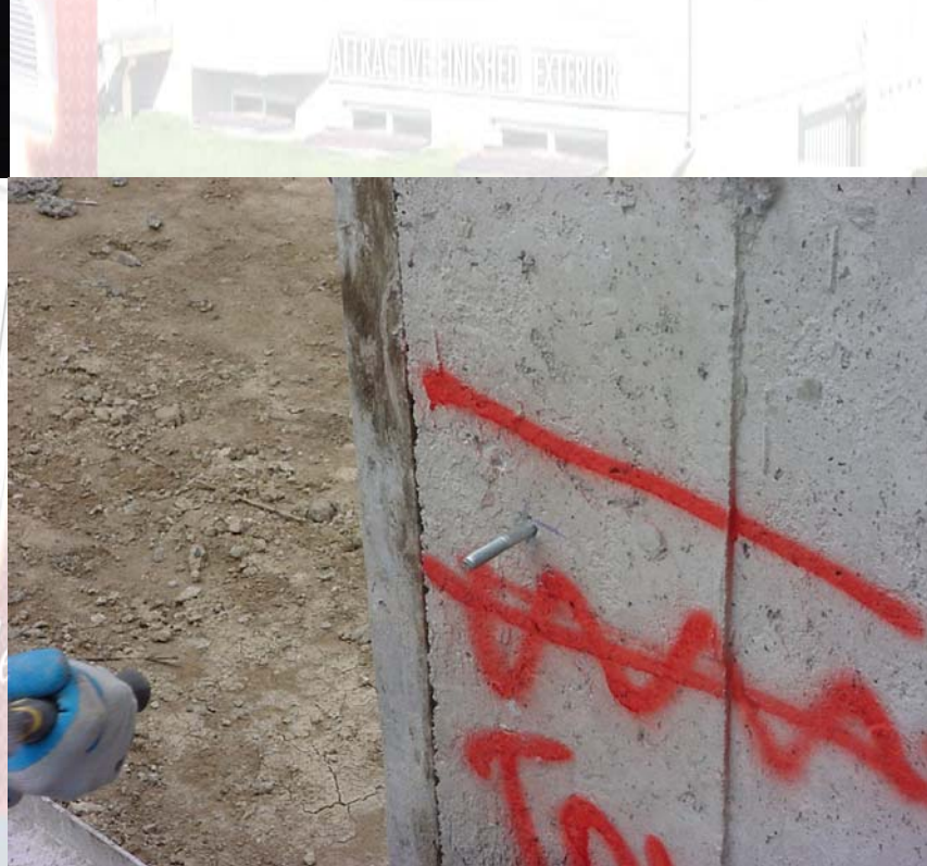
Well anchors pre-installed
