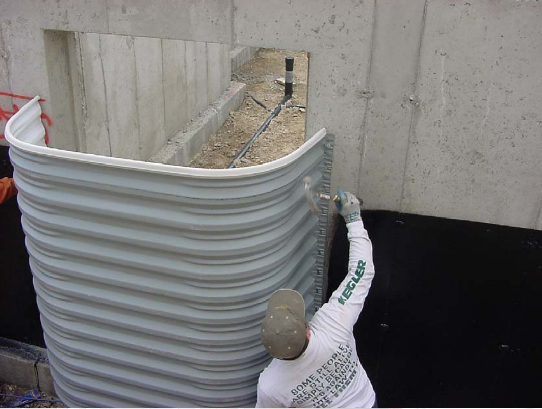
Well anchors pre-installed
